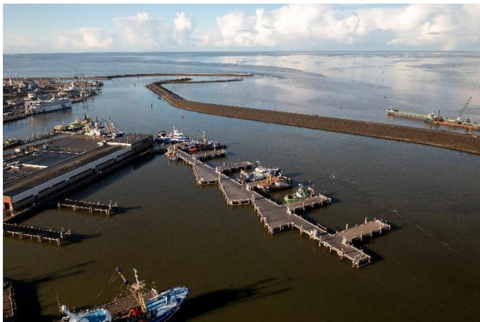
Zaagtandsteiger (Sawtooth pier) in the fishery port. Photo: Joachim de Ruijter
